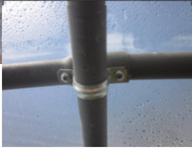
Metal conduit clamp with self-tapping screws
